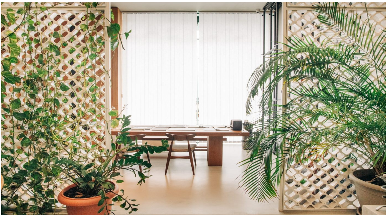
A TERRAZZO GRANITECH FINISH, INSTALLED
